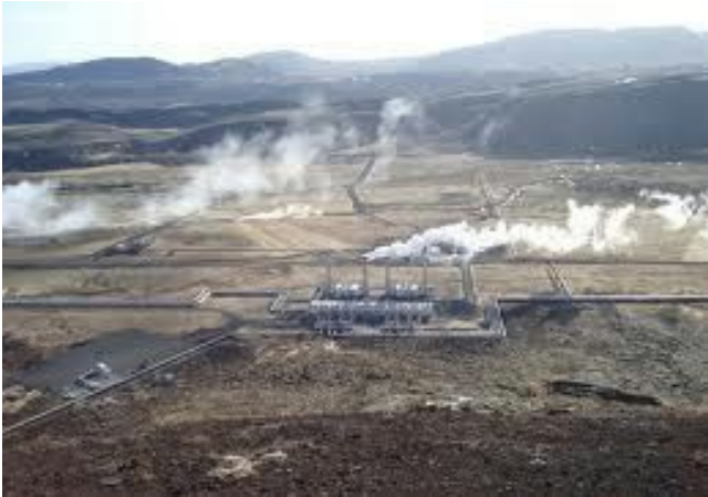
Geothermal Power Plant, Bjarnarflag, Iceland
