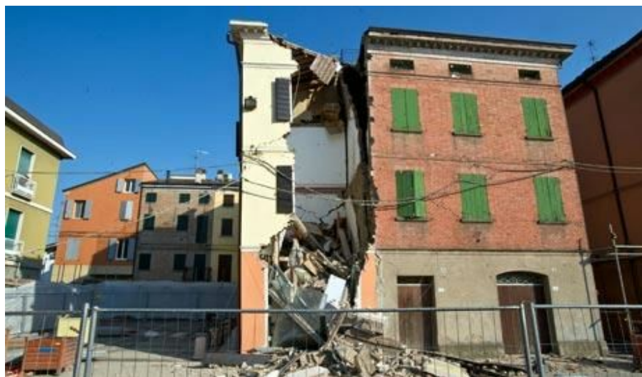
Damaged buildings in Cavezzo, Italy, on Tuesday. The mechanics of earthquakes make accurate predictions unlikely. Photograph: Rex Features
